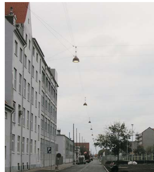
gatelys på wire / streetlight mounted on wire
