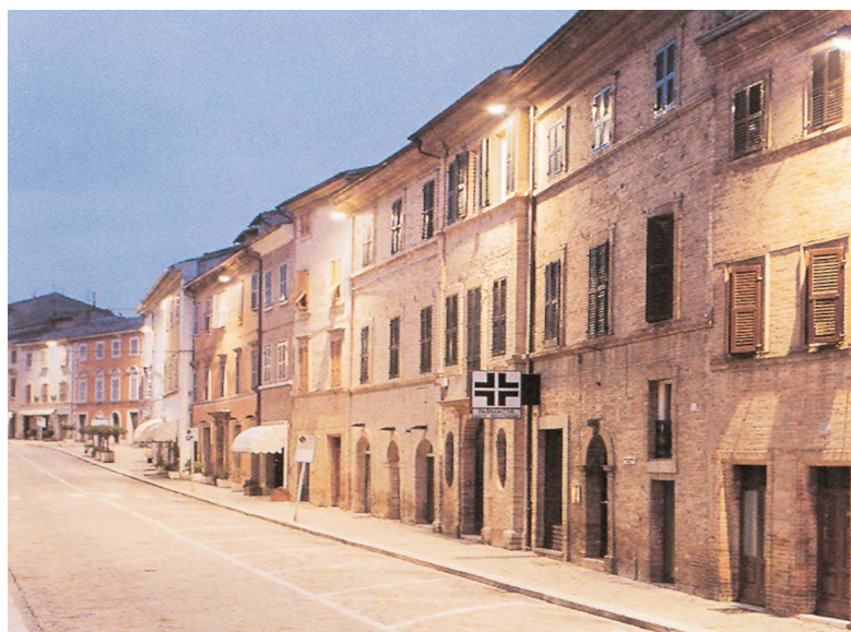
gatelys på bygning / streetlight mounted on building
