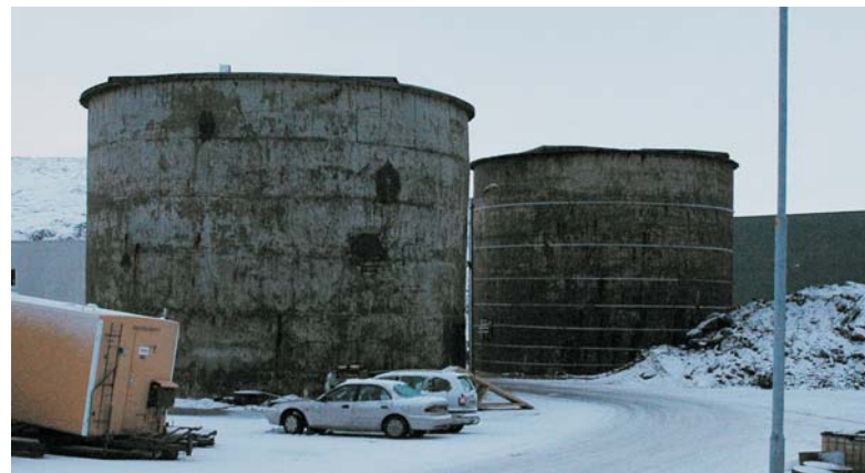
Gamle Salttankene / Old salt tanks
